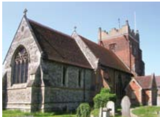
St Mary's Tollesbury. The tower has its origins in the 11th Century. Throughout the church, additions have been made in every century up to the 20th.
